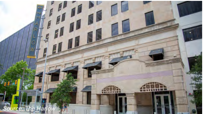
The Harlow is a recent Downtown office conversion, transforming the BancFirst and Medical Arts building into a 265 unit luxury apartment building.
