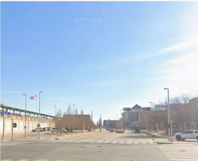
Gaylord Blvd. is currently a major barrier to mobility between Santa Fe Station and Bricktown and points to the west.
