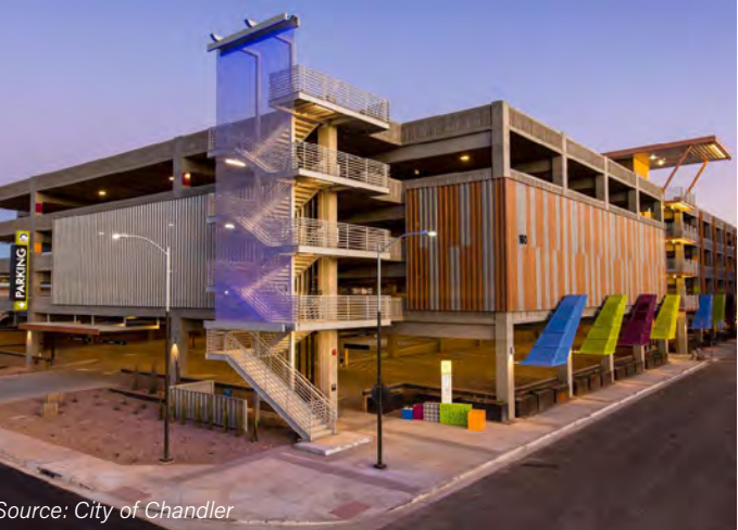
Open-air parking structures and structures not designed to carry the weight of an additional structure are not suitable.
