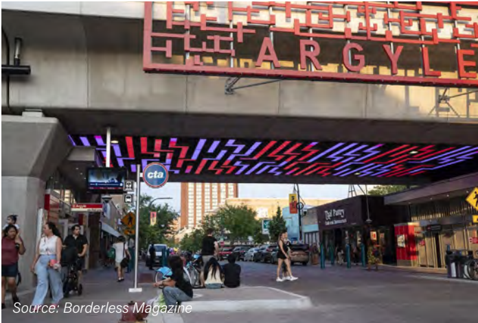
The Argyle Red Line CTA Station in Chicago, IL is an example of a railroad underpass with ample pedestrian space, high quality art and lighting, and adjacent retail that activates the experience.
