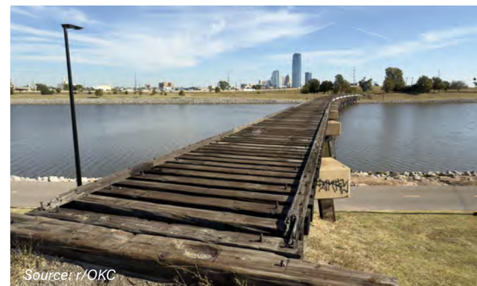
An existing historic railroad bridge is being reconstructed as a pedestrian bridge, which will enhance mobility around and along the river.
