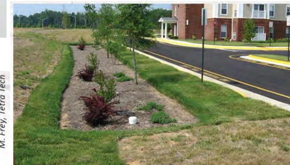
Stormwater infiltration trench, Stafford County, Virginia
