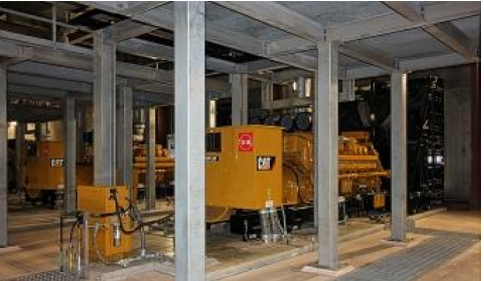
The Draper Water Treatment Plant was knocked off-line during the May 2013 tornado resulting in residents and businesses being unable to use water as crews worked to restore electricity to the plant. Emergency Generators, funded by Federal Disaster Recovery Grants, were installed at the plant to ensure uninterrupted water service in the future.
