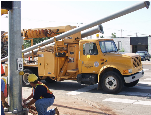
Council Priority: Focus on Infrastructure
